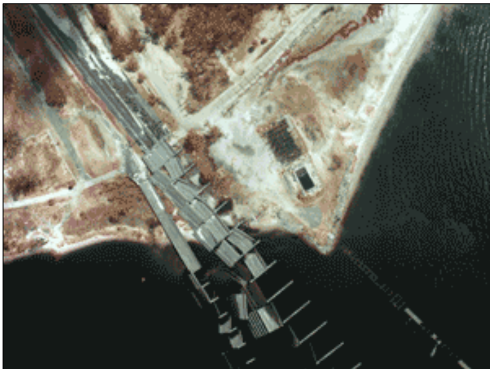
Figure 1 – Roadway damaged by hurricane Katrina Source: NASA (2005)
