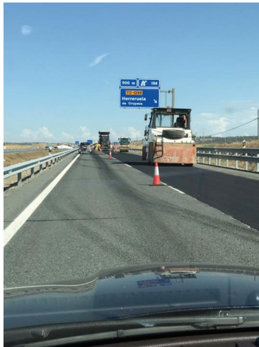
Image 2: Resurfacing works (Source: AEC).
