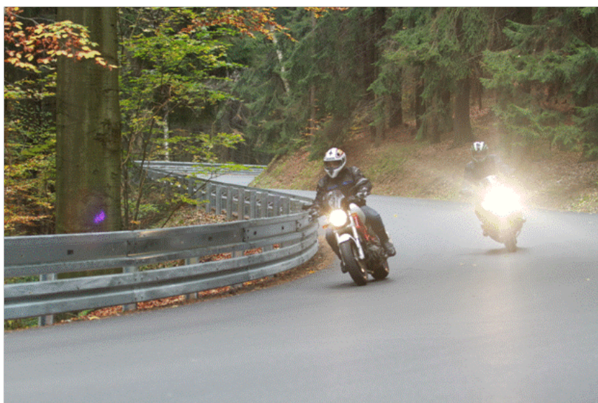
Figure 1: A motorcyclist-friendly safety barrier manufactured by ArcelorMittal Ostrava is equipped with the lower guard strip that saves motorcyclists from severe injuries
